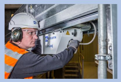
"As well as being more robust, the KilnLoq<sup>®</sup> gives the plant a much better oxygen, CO reading that they can then use to optimise the kiln, by balancing the air flow split between kiln / calciner, which will also help to reduce fuel consumption," explains Sathish. "It's a relatively small project that can have a very big impact."
